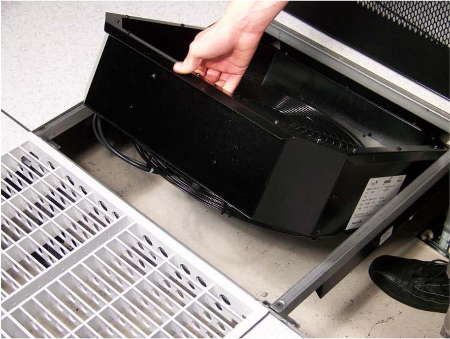
Figure 10 - Installation of Fan Unit onto Tool Less Hangers
