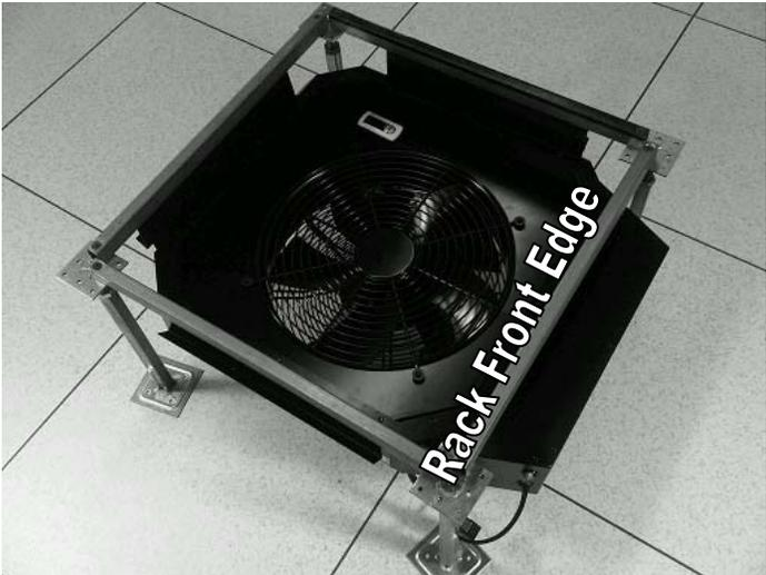
Figure 9 - PowerAire™ Unit Installed on hangers in correct orientation
