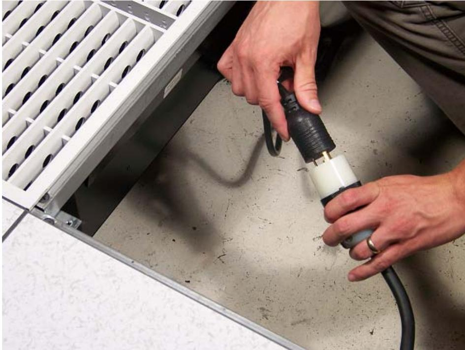
Figure 17 - Connecting power to the unit
