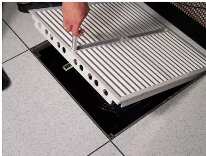
Figure 20 - Installation of DirectAire Panel
